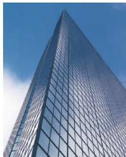
HVAC / Building management
